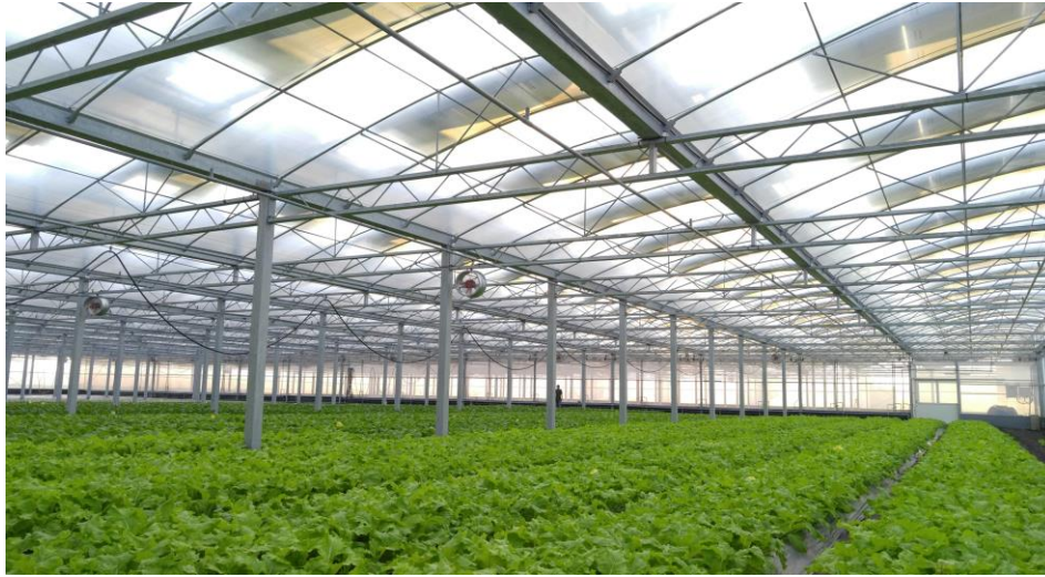
Photos 1~3: GES' award winning 1MW project in Fangliao, Pintung County, Taiwan
